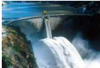
Hydro Power Plants
